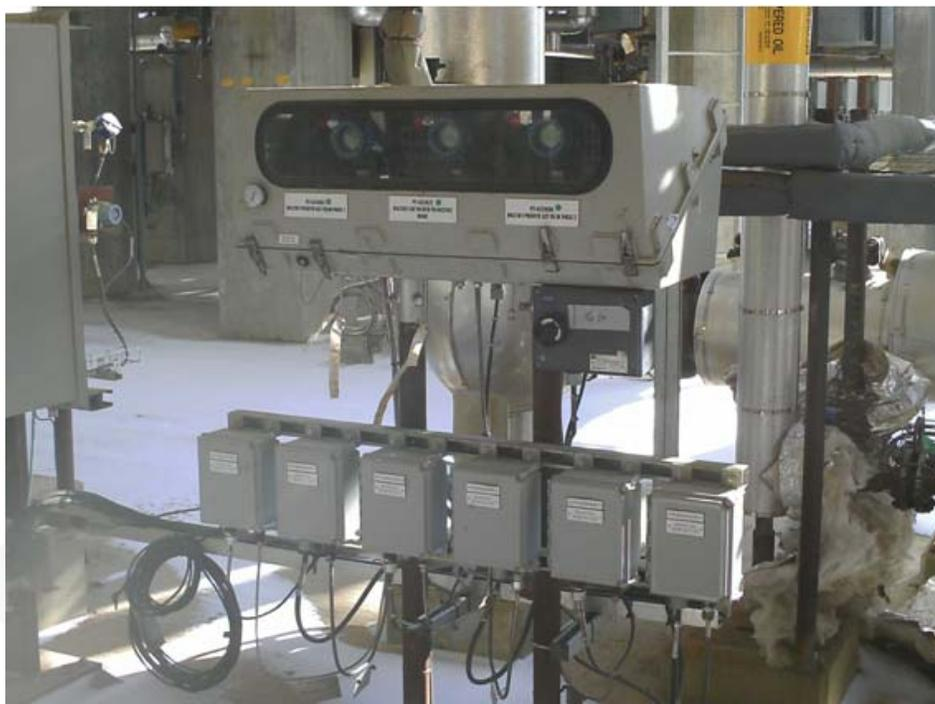
Above: Three pressure transmitters mounted in one instrument enclosure with a series of enclosure heater circuits below. By observing the transmitter body temperatures via the HART signal, Shell can detect a heater circuit fail from a low body temperature.
