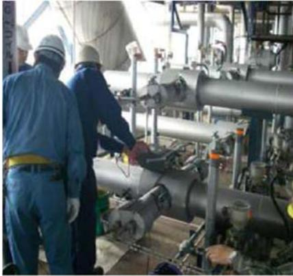
After installing a conditioning orifice plate, flow signal stability was verified. This in turn provided an accurate measurement for improved plant availability and greater throughput.
